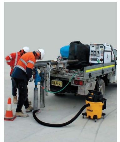
PPB-8-15-AU Concrete Coring
