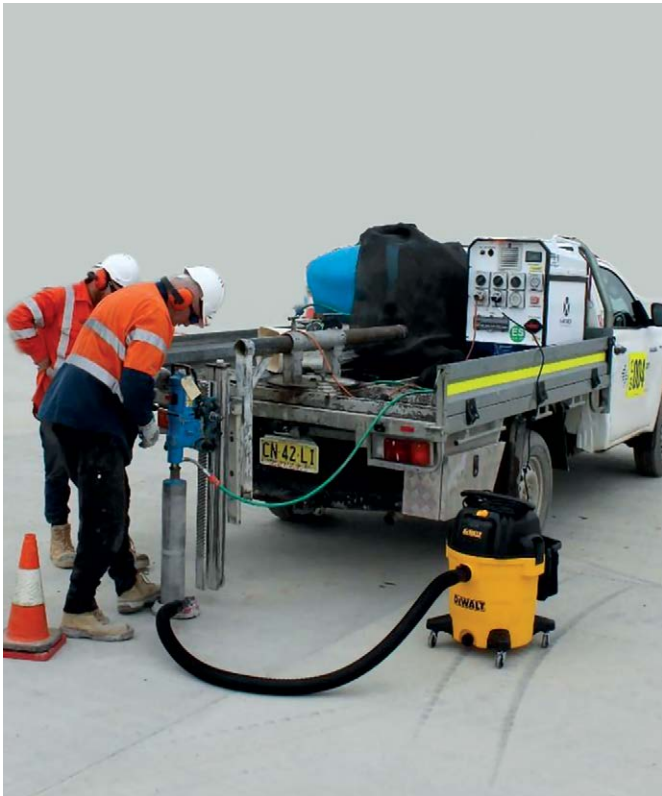
PPB 8-15 Concrete Coring
